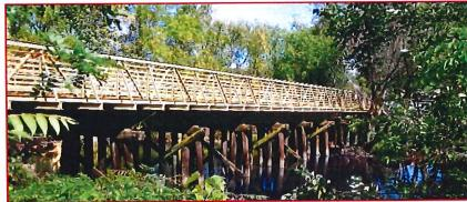
Design, construction engineering and right-of-way acquisition services for 1.62 miles of a multi-use path along the Kalamazoo River in the City of Albion. This MDOT Enhancement Project included a minimum 10 ft.-wide concrete trail along residential areas and HMA trail at all other locations. The project also contained three 14 ft. clear pedestrian bridges, including the utilization of an abandoned 270 ft. railroad trestle.
